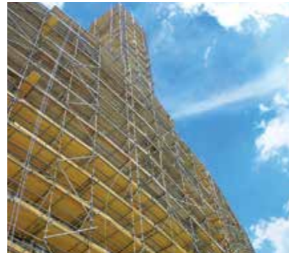
Project : Bright Star Tower, Sheikh Zayed Road Client : Dubai Contracting Company Location : Dubai Scope : Access scaffolding to erect cladding from
